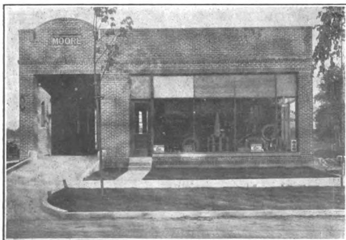
Garage and salesroom of the W. C. Moore Auto Company, which has just been completed at Wilkes-Barre, Penna.
